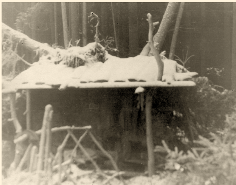
In remote, hard-to-reach areas — most often on islands in marshes — the partisans did not build underground bunkers, but rather small, well-camouflaged above-ground huts.
